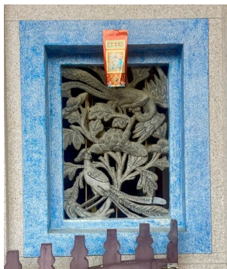
Photo 3: A fretwork window panel made by stone. (Photo taken by the author, September 2022)
